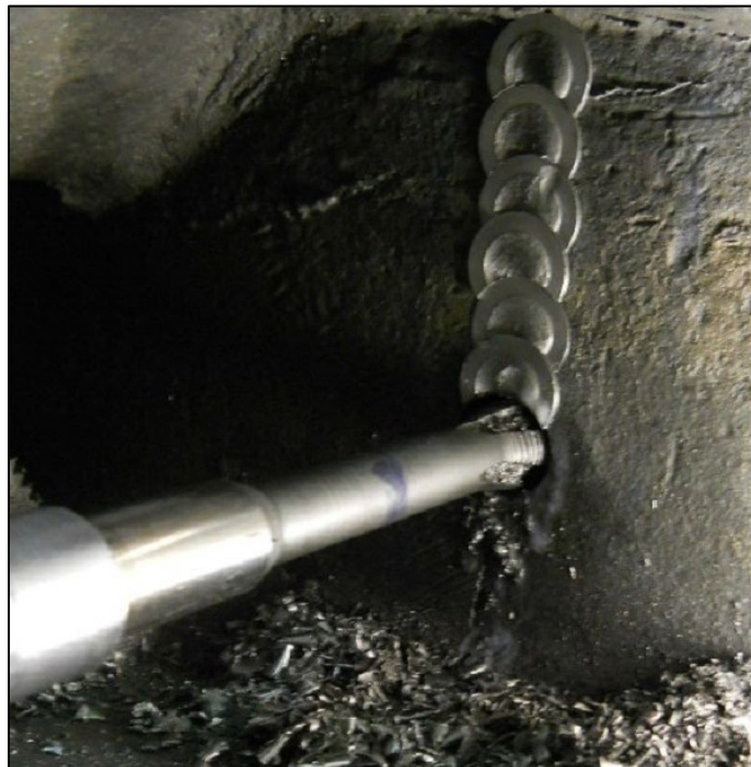
Figure 3: The QuantiServ Metal Stitching Process [14].
