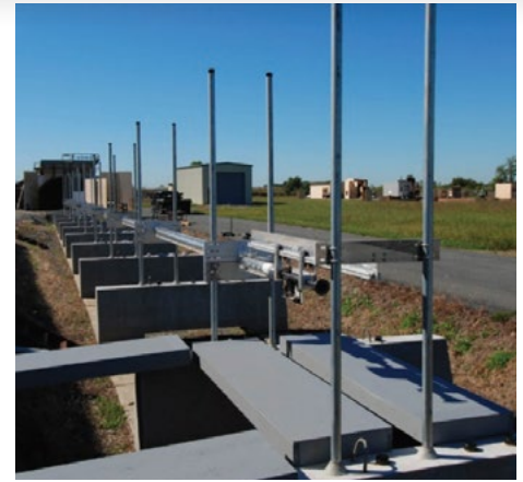
Figure 7: Dynamic RPG Firing Facility (Photo Courtesy of ARL).
