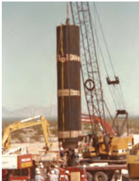
Figure 2: Launch Tube Being Emplaced for Test.
